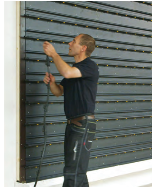
Natural Greenwalls® rails are mounted, drip hoses are inserted and finished with fittings.
