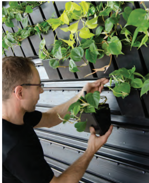
Natural Greenwalls® pots are clicked into the rails.
